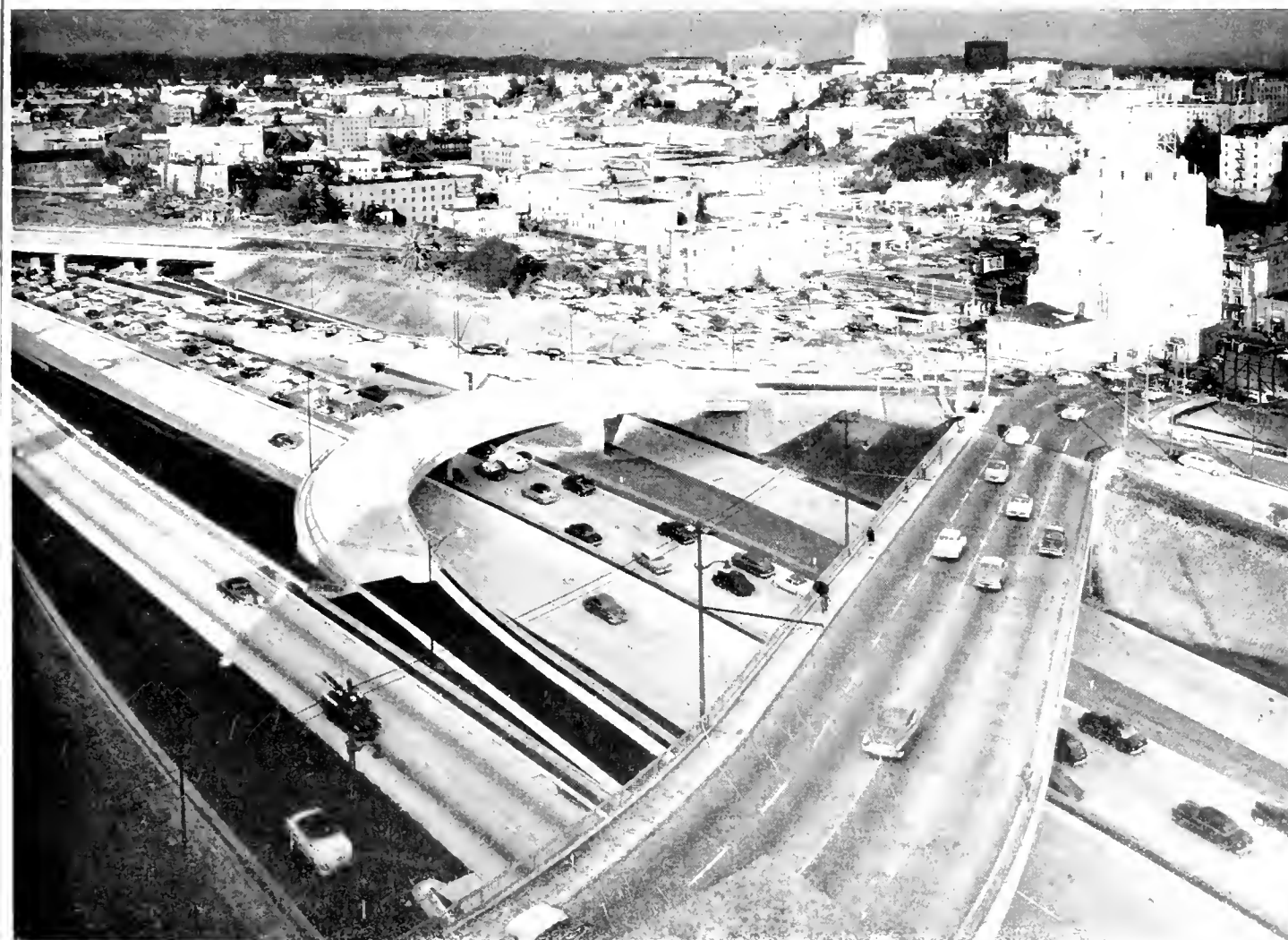
Evening peak hour traffic on the Harbor Freeway, with the Fifth Street Overcrossing in the foreground, the Fifth Street southbound on-ramp in the center and the northbound on-ramp carrying traffic in the direction of the four-level structure
